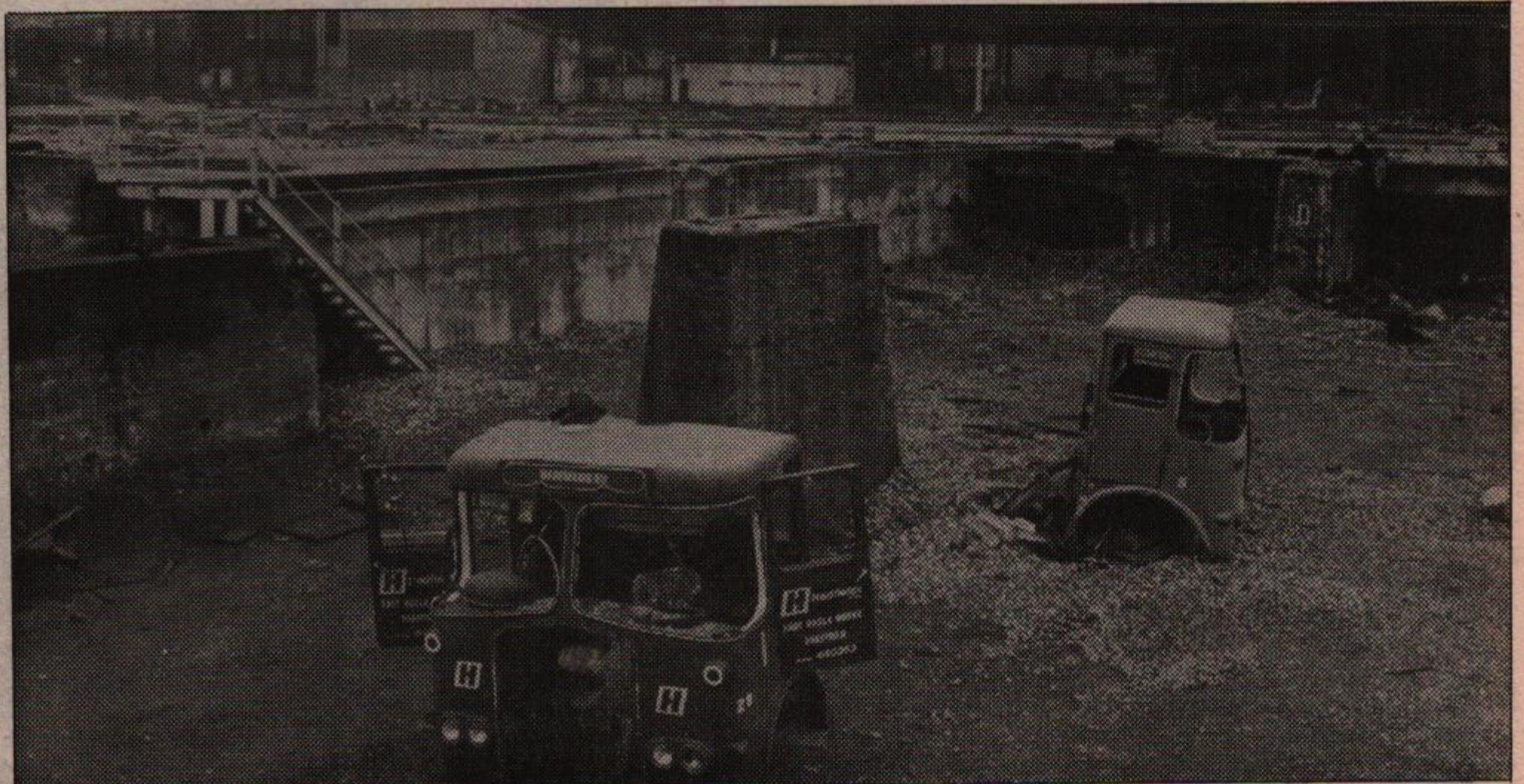
A rundown steel factory in Sheffield.
